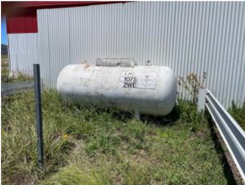
Figure 3: Existing above ground LPG Tank
