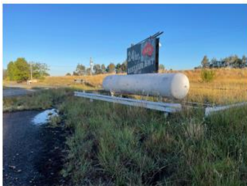
Figure 5: Existing above ground LPG Tank
